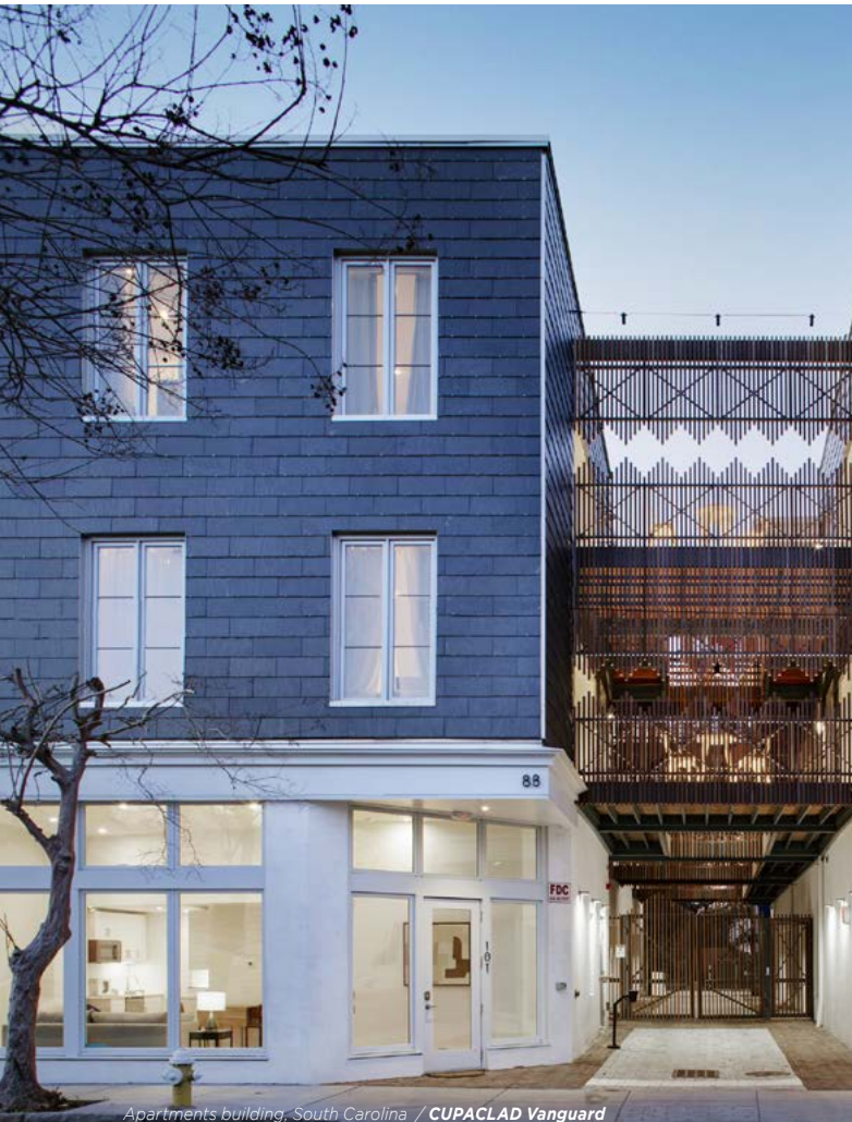
Apartments building, South Carolina / CUPACLAD Vanguard
